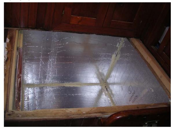
Here is the same space with the inner layer of ½" foam, and the pultruded fiberglass panels that are the liner of the refrigerated space glued in place and sealed up with epoxy resin with easy sanding fairing mixture in it.
