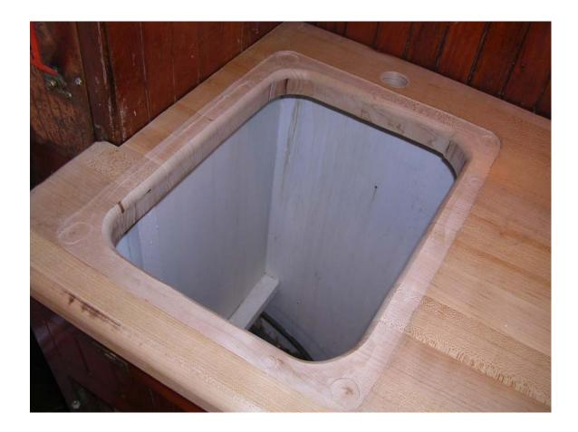
Here is the sink after cutting off its flange and securing bolts, and evening everything out best I could. I trusted to make this a tight fit and seal it up with Sikaflex 291, thinking that would be adequate to hold the sink in place. That didn't work, as the sink has pulled up slightly from the counter-top and is going to have to be rebedded after I figure out how to hold it down in its place more firmly.
