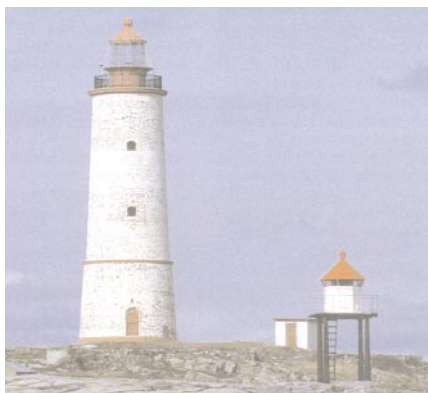
Indre Torungen Light Tower (disused)
