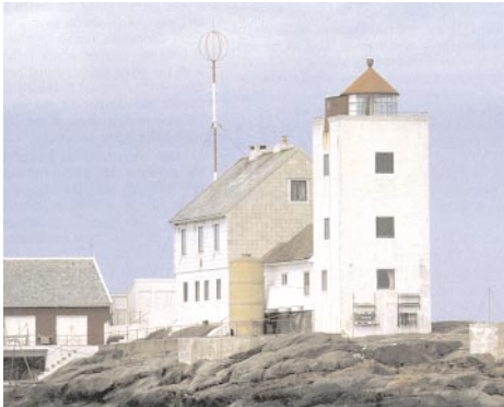
Fulehu Disused Lighthouse
