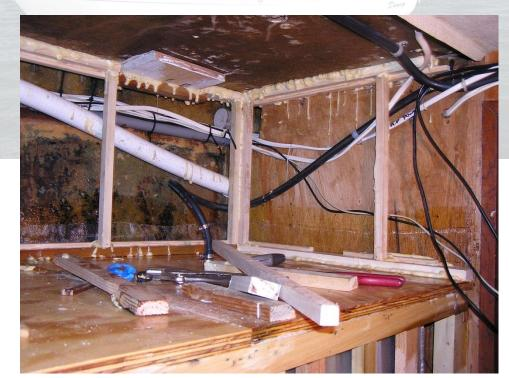
Building the enclosure here required rerouting the deck drains, some tank vents, and some wiring. Below is the unit installed and operational, but not enclosed.
