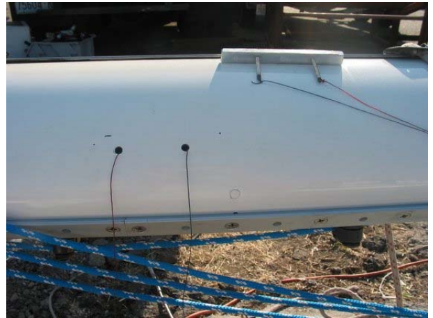
Figure 7. The twine now runs inside the mast from the backing plate to the mounting holes.
